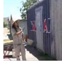
Stucco on a Shipping Container
