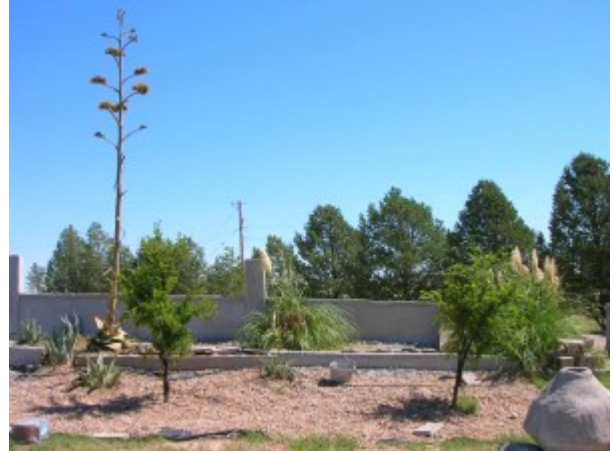
Another view of the surface bonded block wall.
