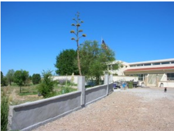
The concrete block wall before surface bonded cement is applied.
