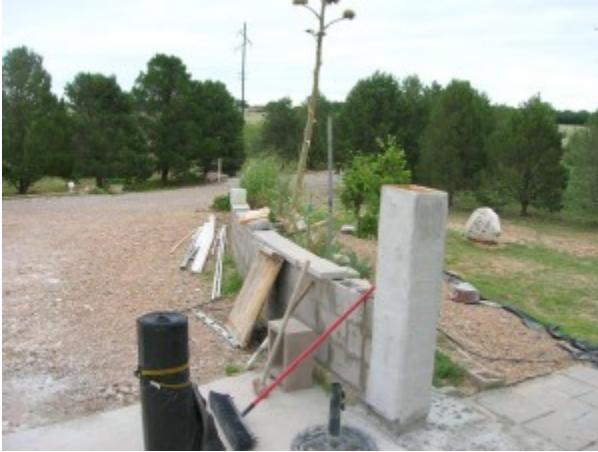
The concrete block wall before surface bonded cement is applied.
